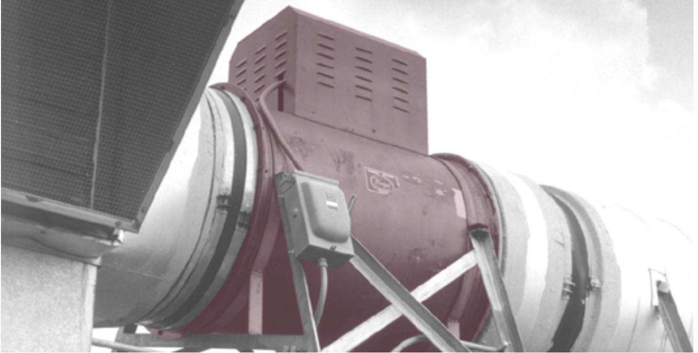
Horizontal, roof-mounted, belt drive Duct Axial® fan performs integral function in heat recovery system.
