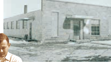
The first factory. 1947
