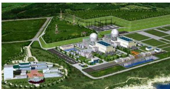
SHIN-KORI NUCLEAR POWER PLANT UNIT NO. 3,4
