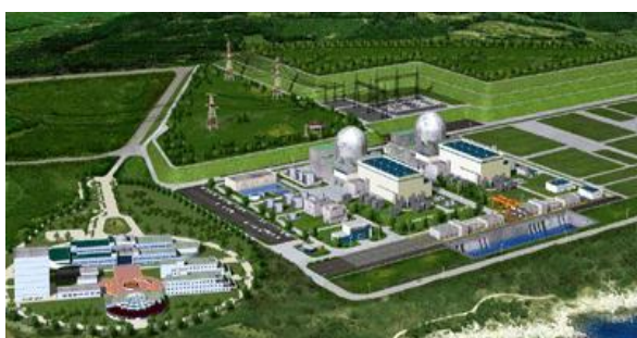
SHIN-KORI NUCLEAR POWER PLANT UNIT NO. 3,4
