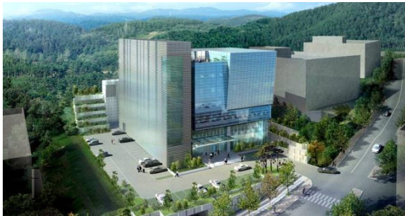
Dongbu hwajae Data Center
