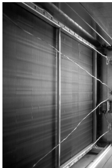
Figure 24. Low-limit sensor
