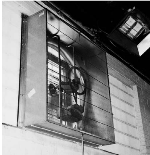
Fan shown mounted in wall
