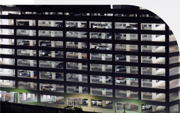
OPEN CAR PARK
