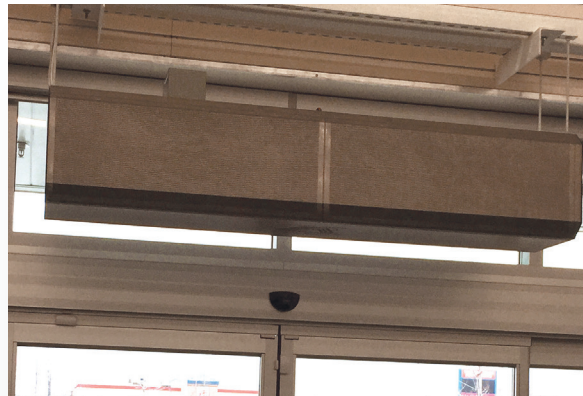
Model CED | Top Mount (Threaded Rods)
