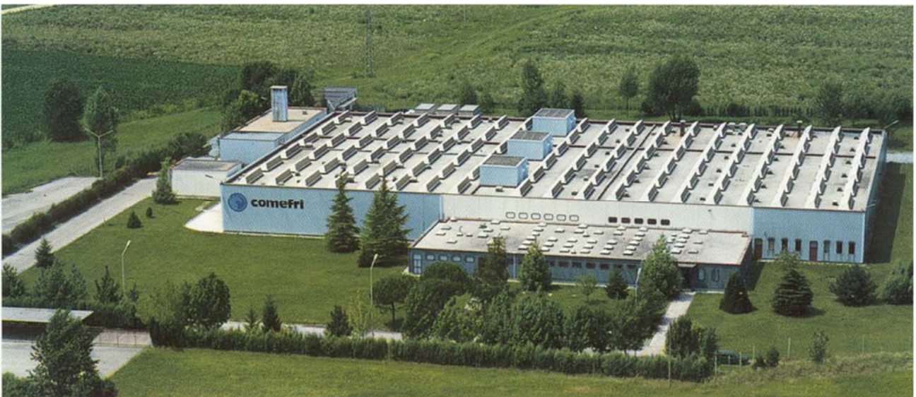
COMEFRI SpA factory at Artegna (UD) – Italy with 6.300 m 2 workshop. Production of industrial fans and special executions.
