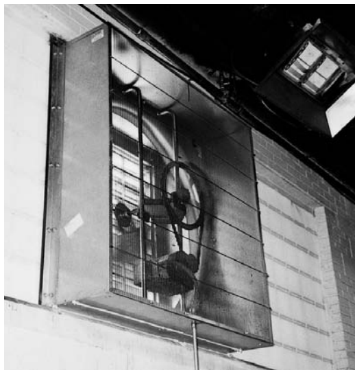
Fan shown mounted in wall
