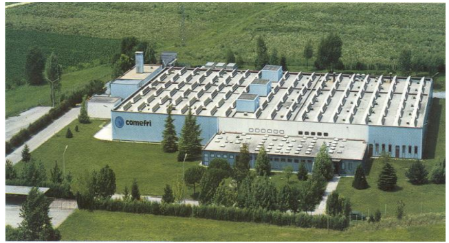
COMEFRI SpA factory at Arterga (UD) – Italy with 6.300 m 2 workshop. Production of industrial fans and special executions.
