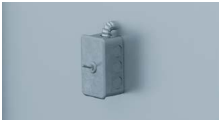
NEMA 1 Disconnect Switch
