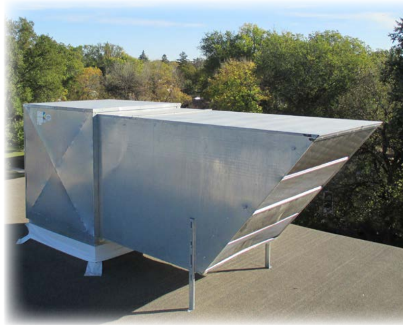
General HVAC Installation
